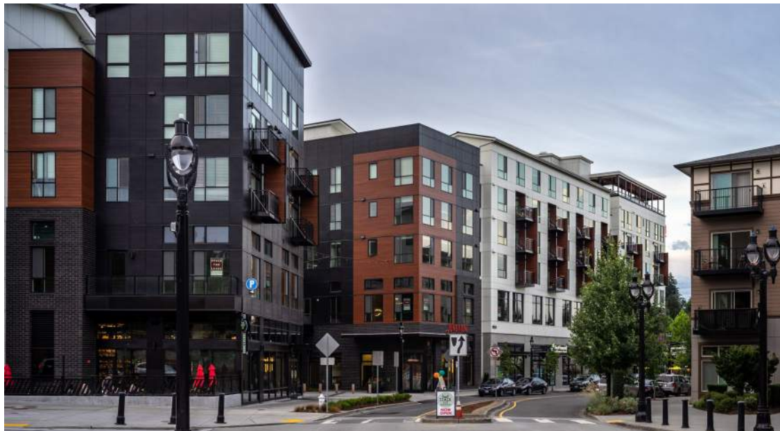
The Junction and Six Oaks, Bothell, WA
