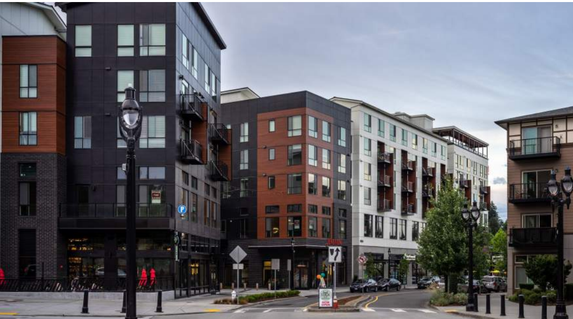
The Junction and Six Oaks, Bothell, WA
