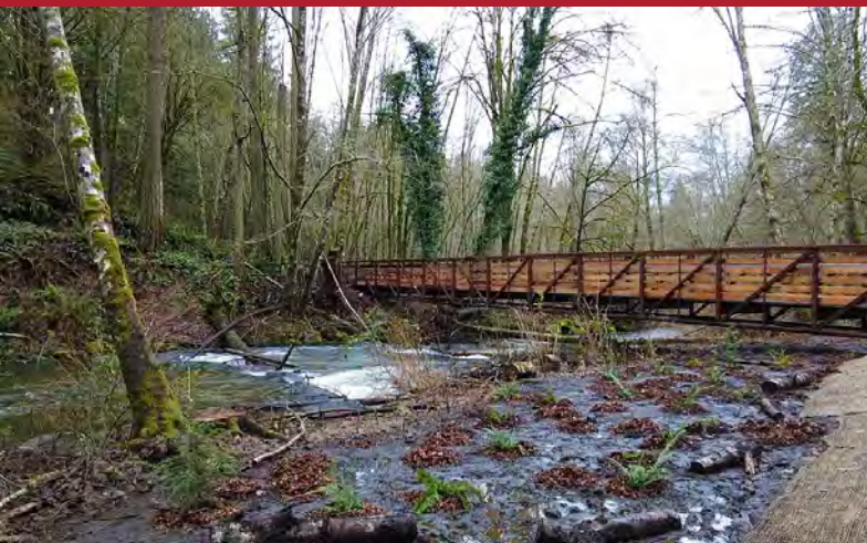
Chambers Creek Bridge Installation- 2021
