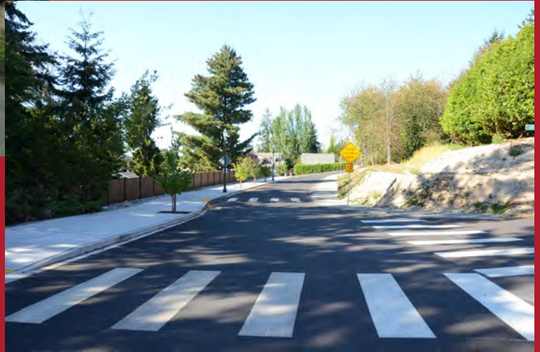
Larsen Lane - 2021 Before & After
