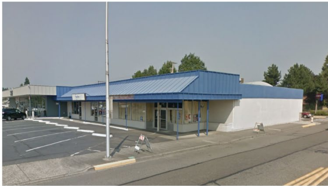
Figure 42. Before / After Facade Improvement Examples in Auburn, WA
