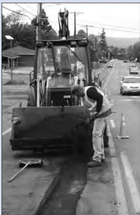
If the cracks are not maintained, they can ravel and increase in size. Unsealed cracks allow water to penetrate into the structure from the pavement surface, which eventually causes potholes and further deterioration. Water intrusion is the number one enemy of pavements.
